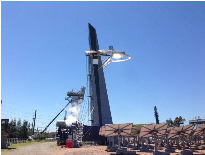
Figure 2 Subcritical steam generation at the CSIRO Newcastle
