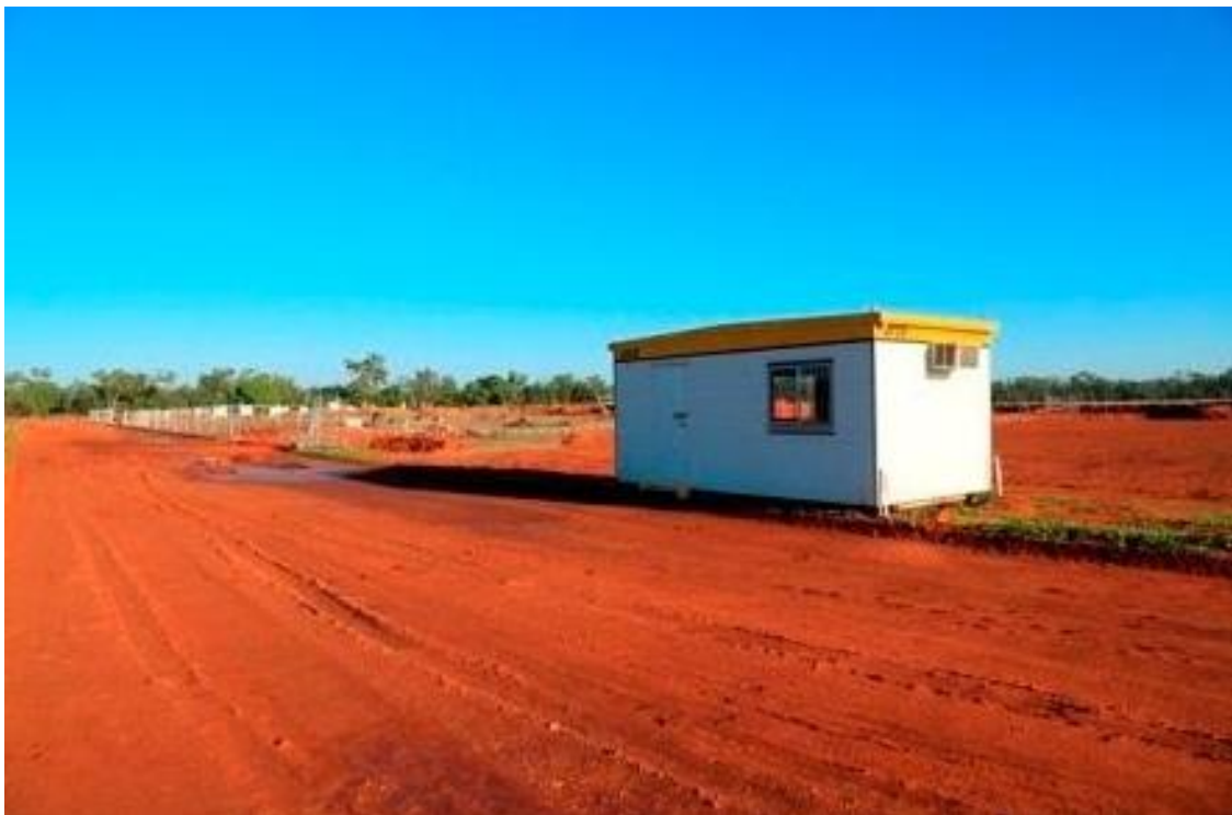
Photo: Project building installation
