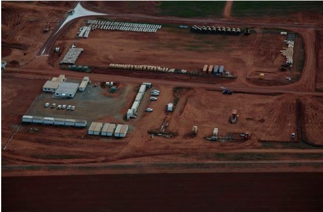
Photo: Early site mobilisation works
