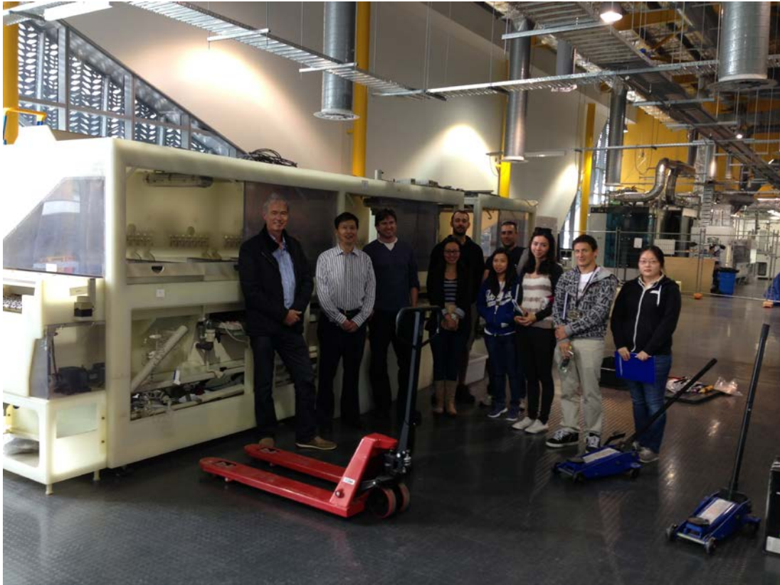
Figure 5: Unique metal plating baths using UNSW technology for the plating of solar cell contacts designed by world expert Dr Ji. These have been constructed in China by the company Kuttler and now installed in SIRF at UNSW.
