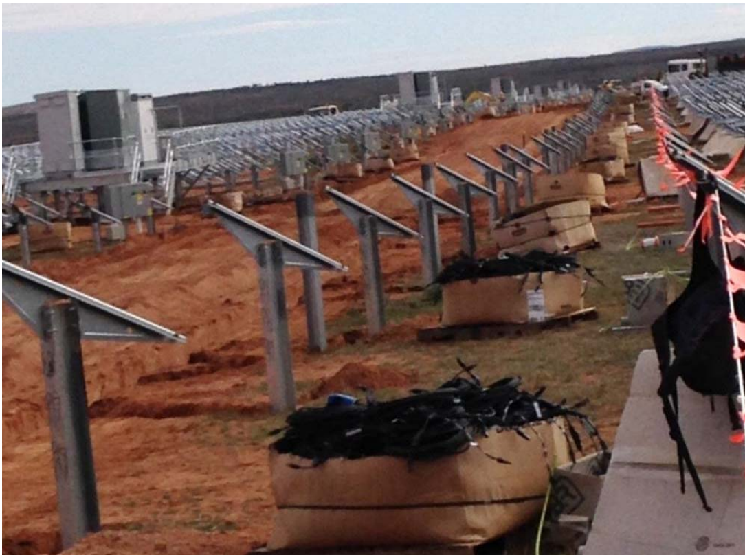
Photo: Pre-staging of harnesses to the work area
