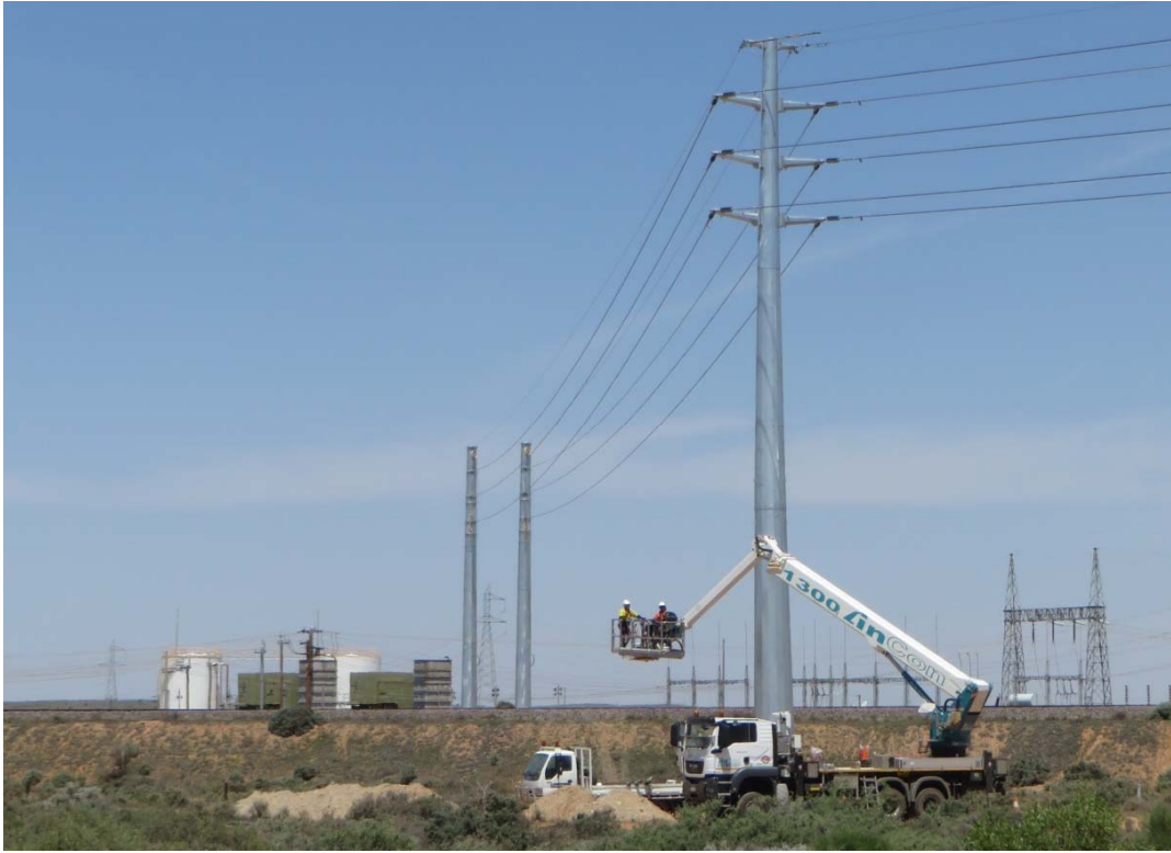
Photo: New 22kV lines crossing over the railway at Broken Hill
