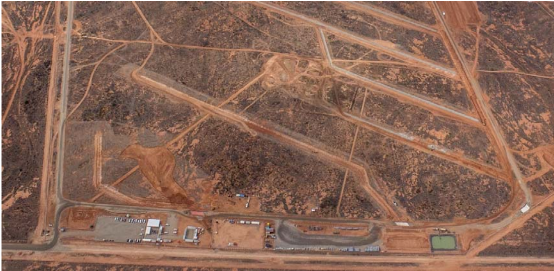
PHOTO: Aerial photograph showing different elements of the civil works package.
