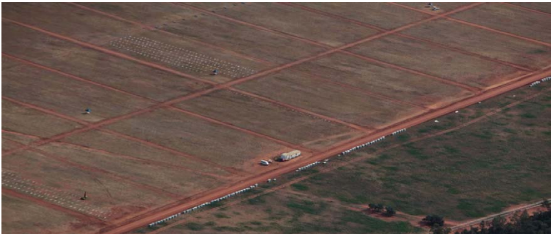
PHOTO: Aerial photo showing staging of posts adjacent to arrays where they will be installed.
