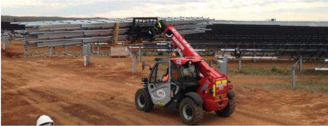
Photo: Pre-staging of end tables to the work area
