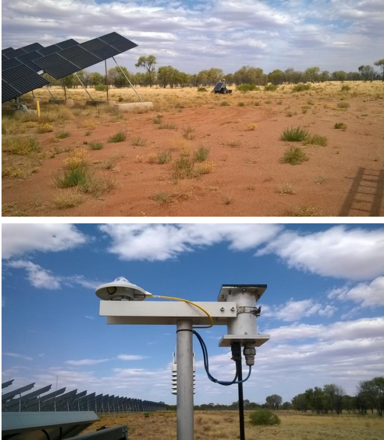
Figure 6: The successful deployment of CloudCAM at Epuron's Uterne site, Alice Springs NT: (top) The CloudCAM system is housed inside a standard 7 x 4 box trailer containing a sky camera, pyranometer and Vaisala WXT520 for local meteorological measurements; (middle) the placement of the CloudCAM system adjacent to the Uterne solar arrays and (bottom) a close-up showing the optical camera assembly (right of centre) and calibrated Kipp & Zonen SMP11 pyranometer for irradiance validation (left of centre).
