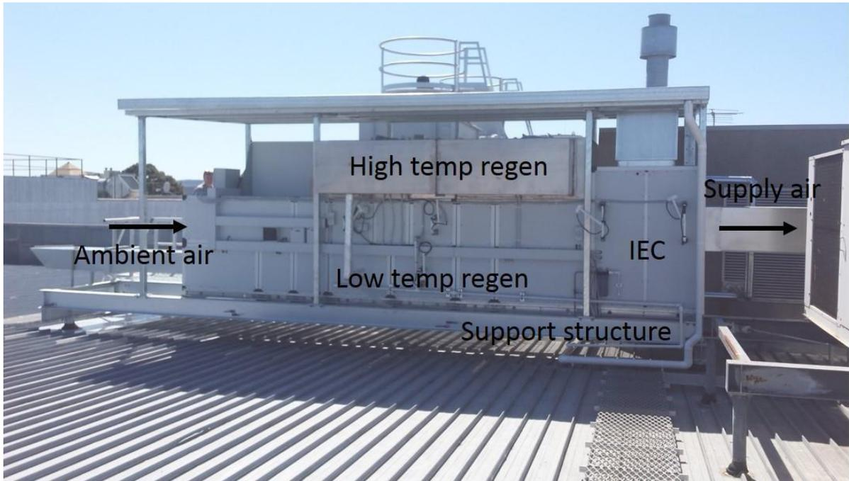
**Figure 3** Two stage desiccant air conditioning system at Stockland Wendouree showing the location of the IEC, and the high and low temperature regeneration paths
