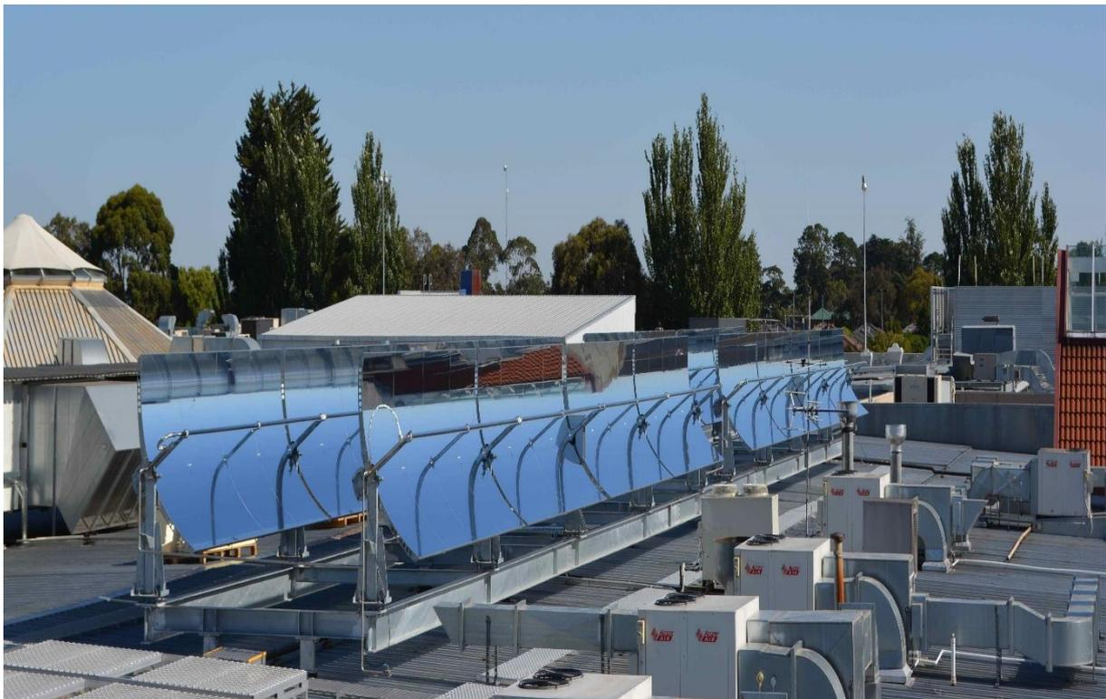
**Figure 2** Parabolic trough collectors installed on the rooftop of the Stockland facility at Wendouree, Victoria
