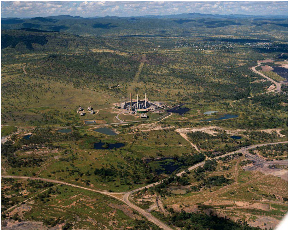
Figure 1: Existing Collinsville Power Station
