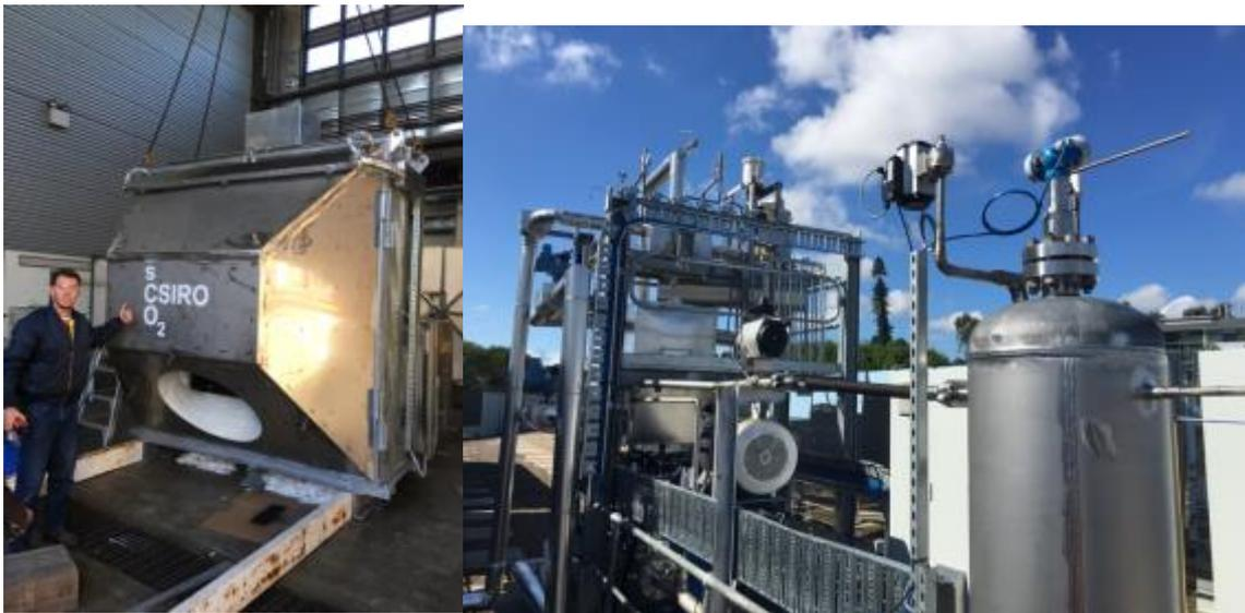
**Figure 1 Completed Solar receiver (LHS) before installation, sCO2 Flow System (RHS)**
