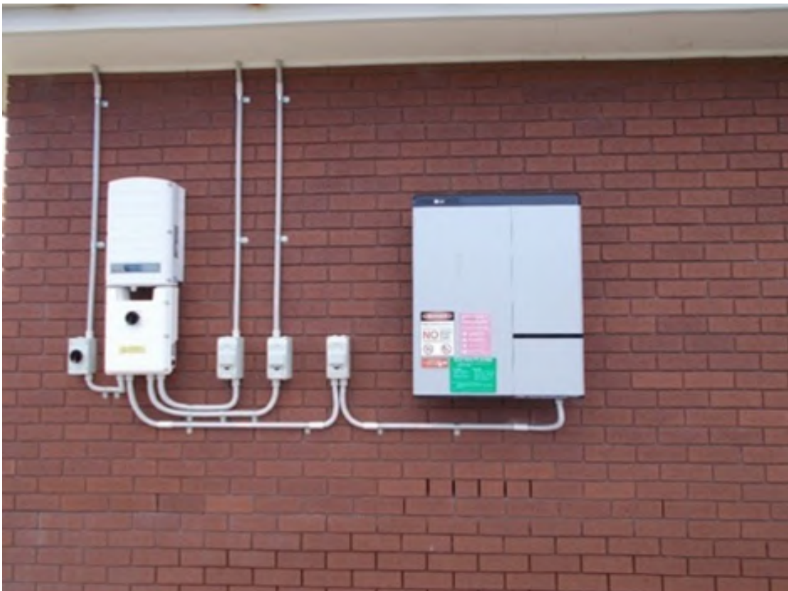
Plate 5: Installation example, external, no enclosure
