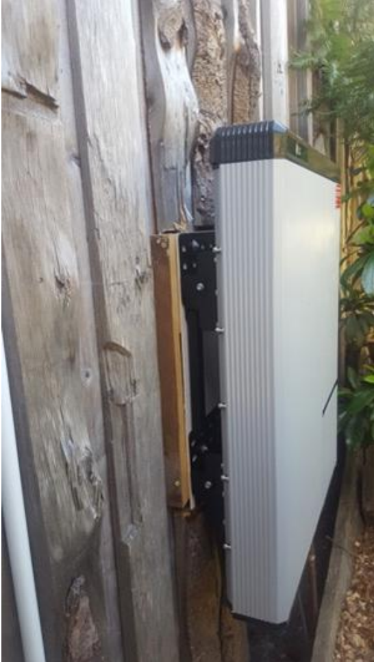
Plate 6: Battery installed behind vegetation (under small eave)
