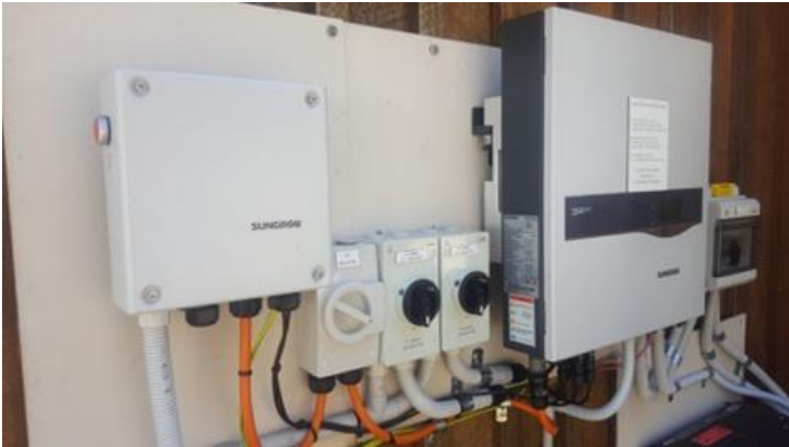
Plate 5: Installation example, external, no enclosure
