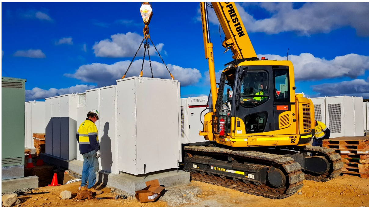
Figure 12 Placing PowerPacks in position
