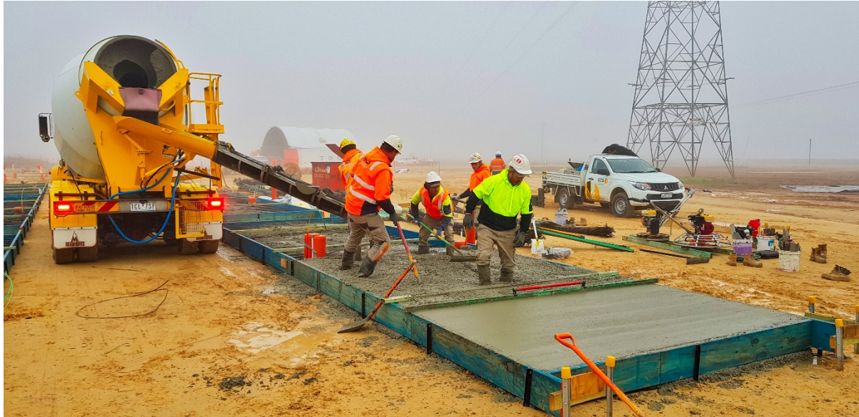
Figure 11 Laying the GESS foundations
