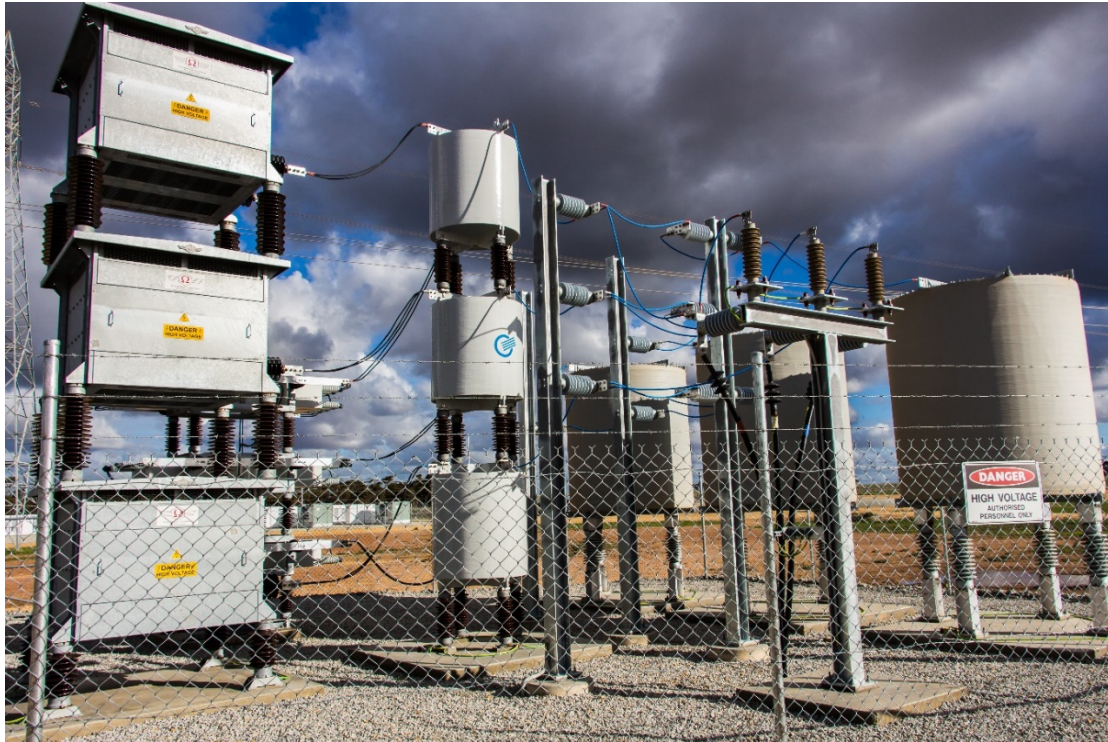
Figure 6 Harmonic filter
