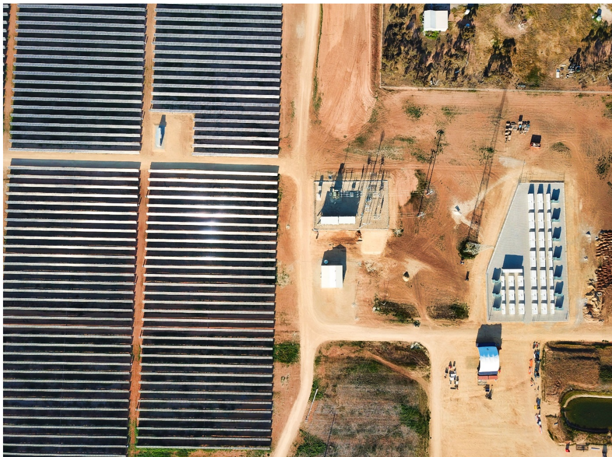
Figure 13 Aerial view of GENSS, GSF, GSF network and the point of connection to Powercor
