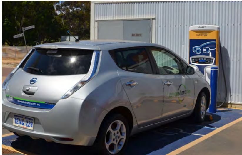
Figure 15 EV charger station and Nissan LEAF at SHAC.
