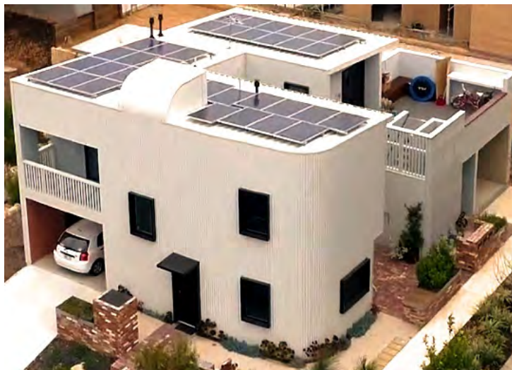
Figure 10 Gen Y solar PV mounted on the roof.
