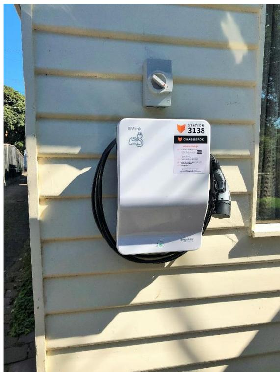
**Figure 2 – First of the trial smart chargers installed at a home in Melbourne**
