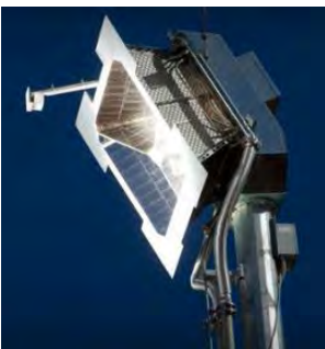
Figure 6.44.2: (left) RayGen's 750 kW p PV power plant in Newbridge, Victoria. Each 250 kW p unit uses a field of heliostats to concentrate sunlight onto a 1 m 2 high efficiency PV receiver. (right) Close-up of a receiver.
