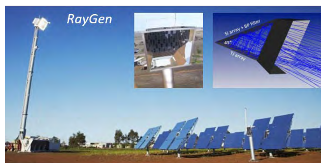
Figure 6.43.1: RayGen's Central Receiver CPV power tower. Inset shows original receiver and V-shaped spectrum splitting receiver design.
