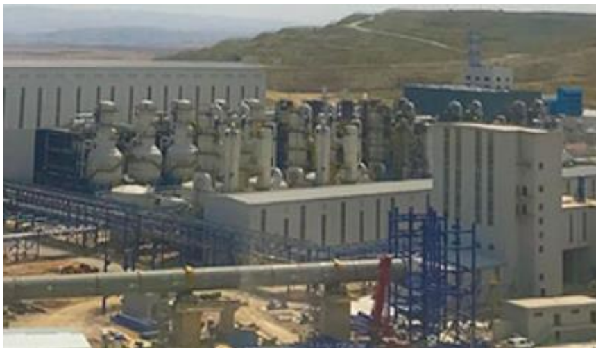
Figure 4 A soda production facility in Turkey. Large falling film and forced circulation evaporators can be seen between the two buildings
