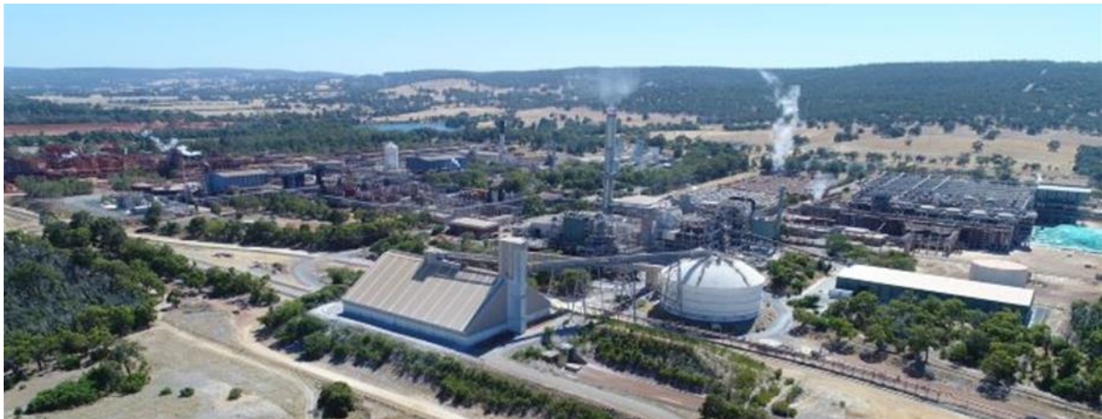
Figure 1 Alcoa's Wagerup alumina refinery, Western Australia
