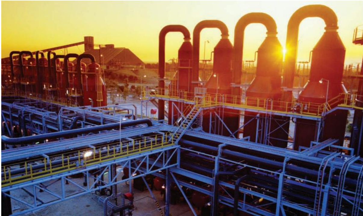
Figure 7 A conventional multi-stage flash evaporation train at Wagerup Flash tanks are clearly visible in the silhouette. Heat exchangers are underneath the flash tanks
