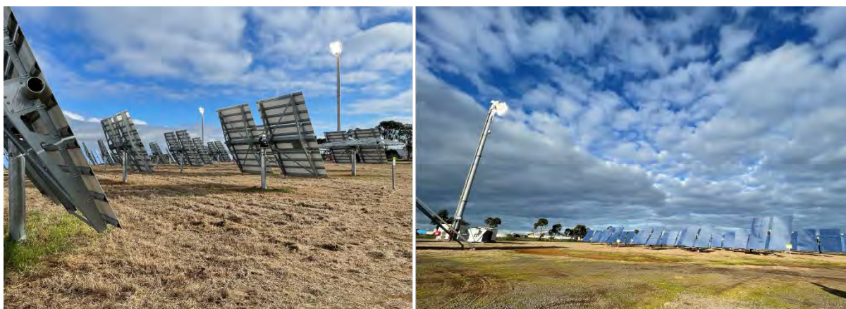
Figure 9. Photos of RayGen's CPV solar farm at Newbridge (Bendigo, Victoria).
