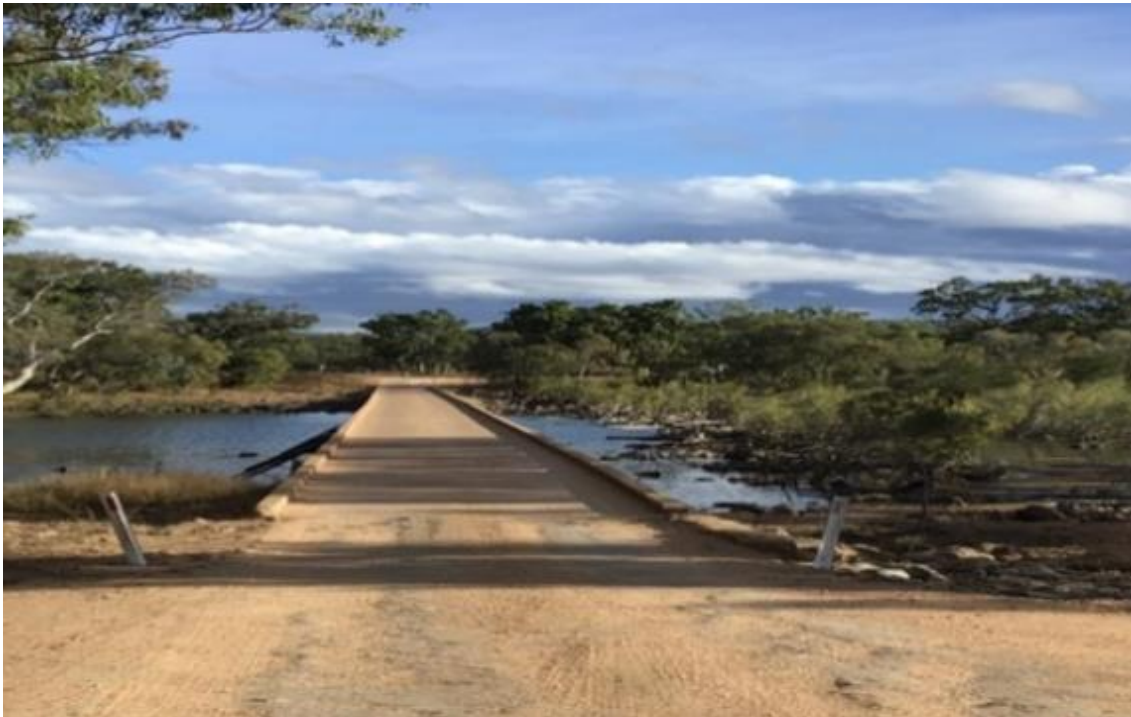
Figure 9: Einasleigh River Bridge on the Gregory Development Road
