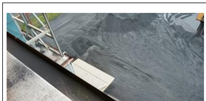
Figure 33– Biochar PCI Plant Coal Yard post first elevation 23/2/23
