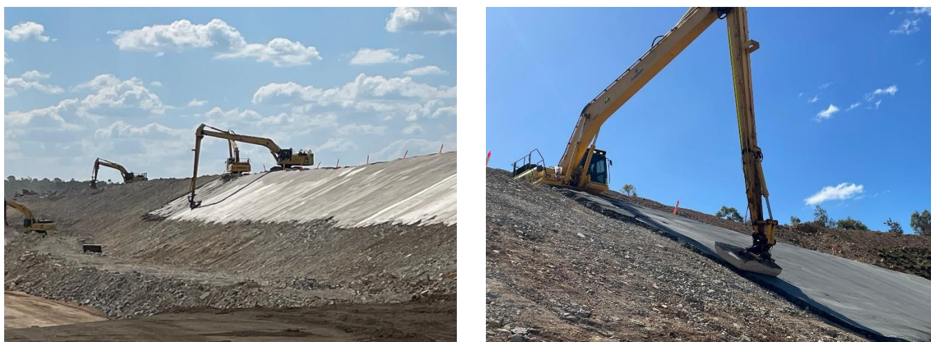
Figure 5: Placement of Cement Screed
