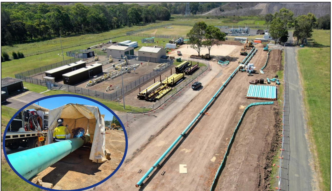
Figure 3: An aerial photograph of the construction of the WSGHH.
