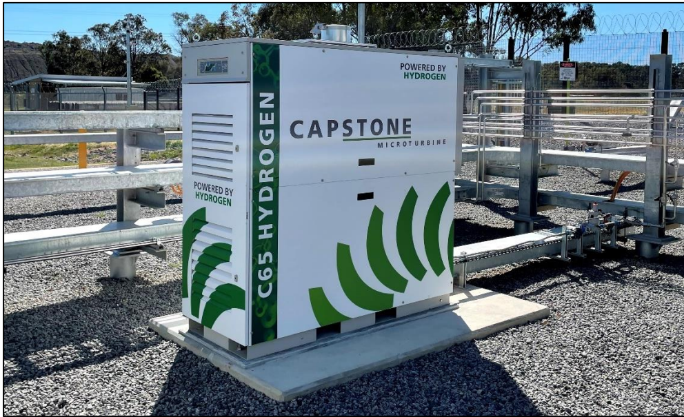
Figure 13: The 65 kW hydrogen micro-turbine at the WSGHH.
