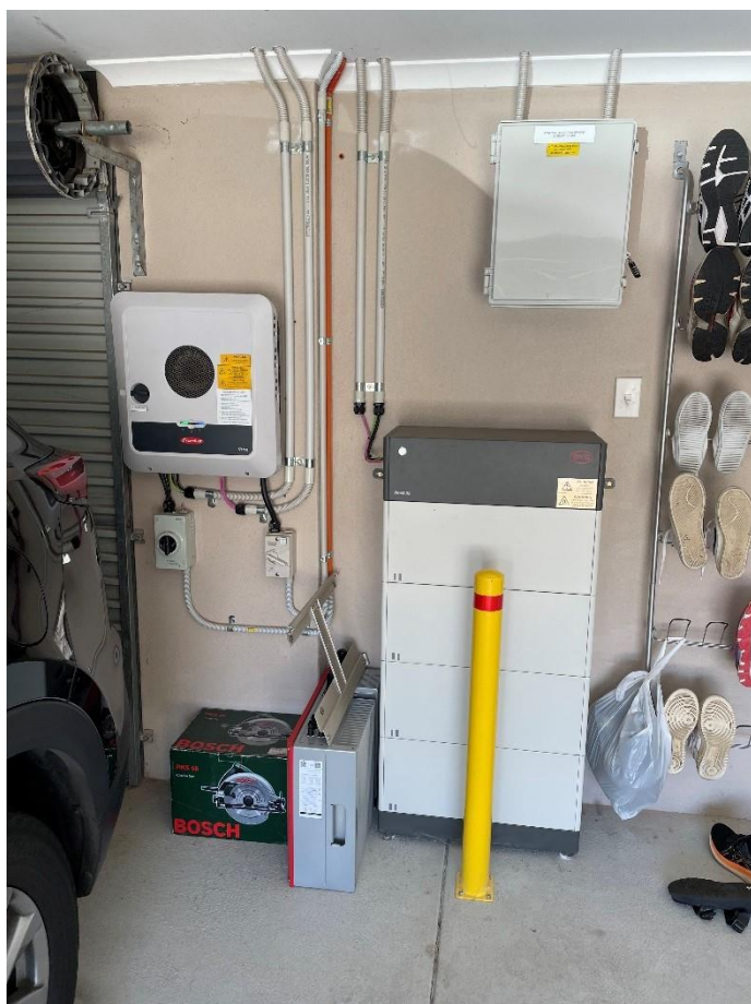
Figure 21: Example of inside garage install with bollard and cabling
