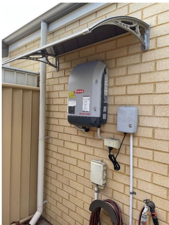
Figure 23: Space constraints led to outside inverters for small number of cases
