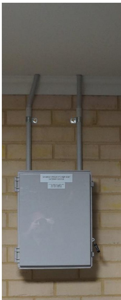
Figure 29: Installed, locked gateway device in garage (PI28)
