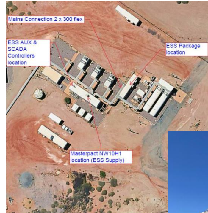
Nullagine Solar Power Station
