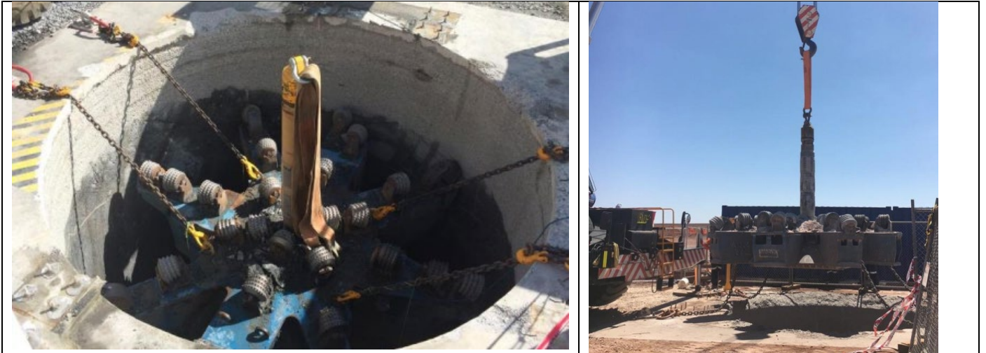
Figure 5: Reamer Head Removal
