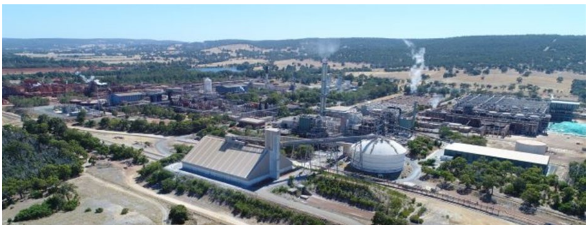
Figure 1 Alcoa's Wagerup alumina refinery, Western Australia
