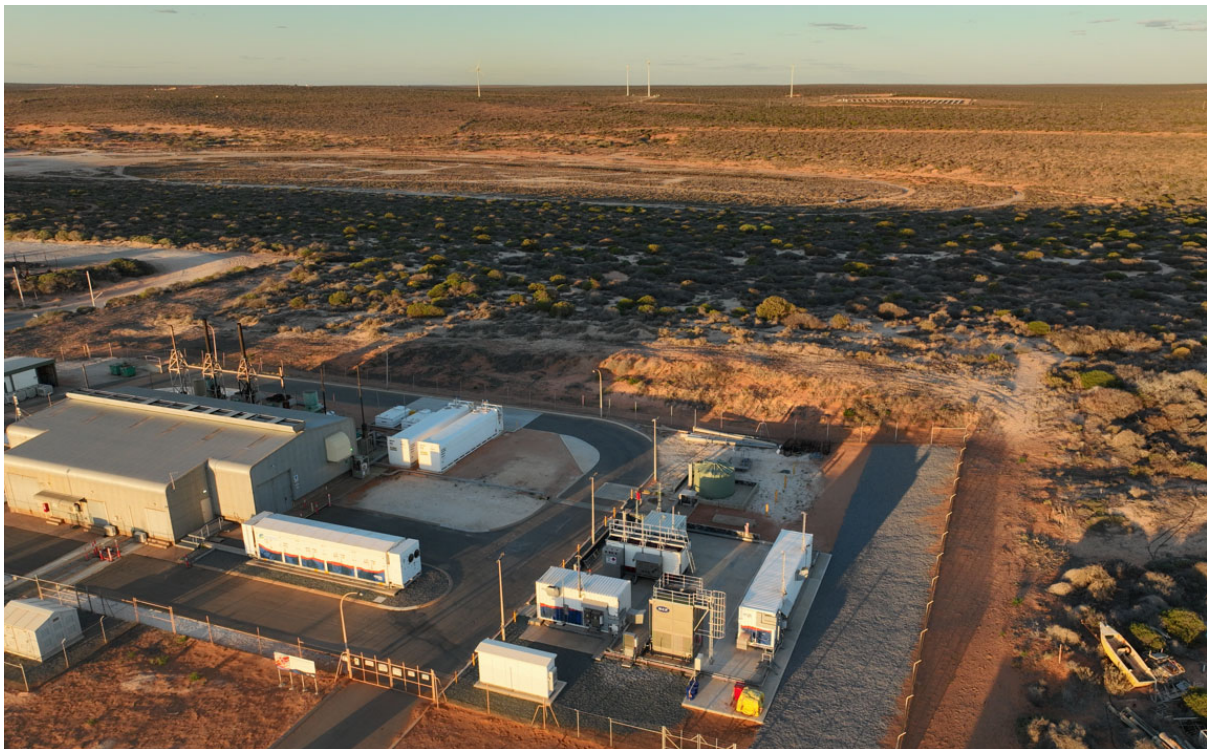
Denham power station and hydrogen plant with the wind and solar farms at the horizon.
