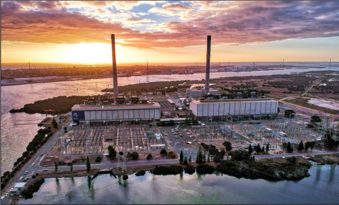
Figure 5 Torrens Island Power Station A (left) and B (right)
