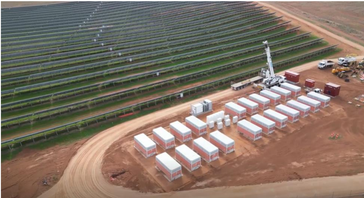
Figure 7: Handling of battery units on site using a crane
